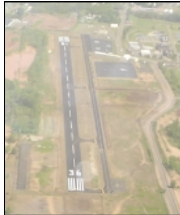
A look at the newly paved runway at MMK. Jim Simmons photo.
